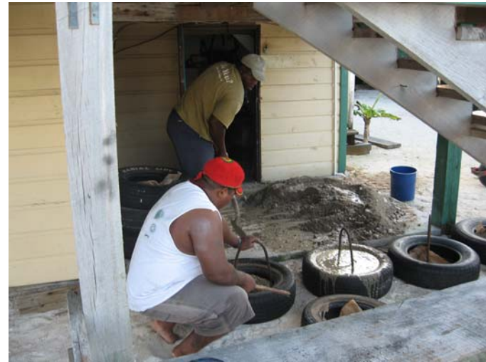
Figure 7. Reserve Staff making anchors for Marker Buoys
